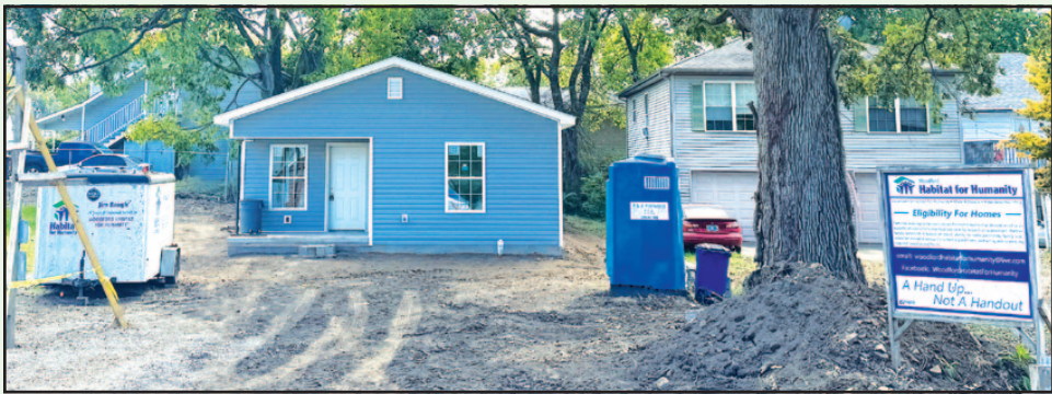
THE NEWEST Habitat for Humanity home being built in Versailles. (Photo by Kennedy Parker)
